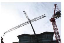
In no time: The WOLFF patented design of the counter jib, pre-assembly of crane components and low initial tower height stand for the fast and economical assembly of the WOLFF 700 in downtown San Francisco. (Source: WOLFFKRAN)
